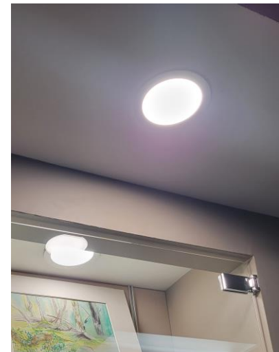
New LED High Hats Installed
