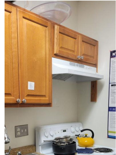
New Range Hood Installed
