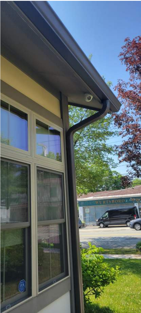
Camera 4 of 8 to be replaced Front entrance of building
