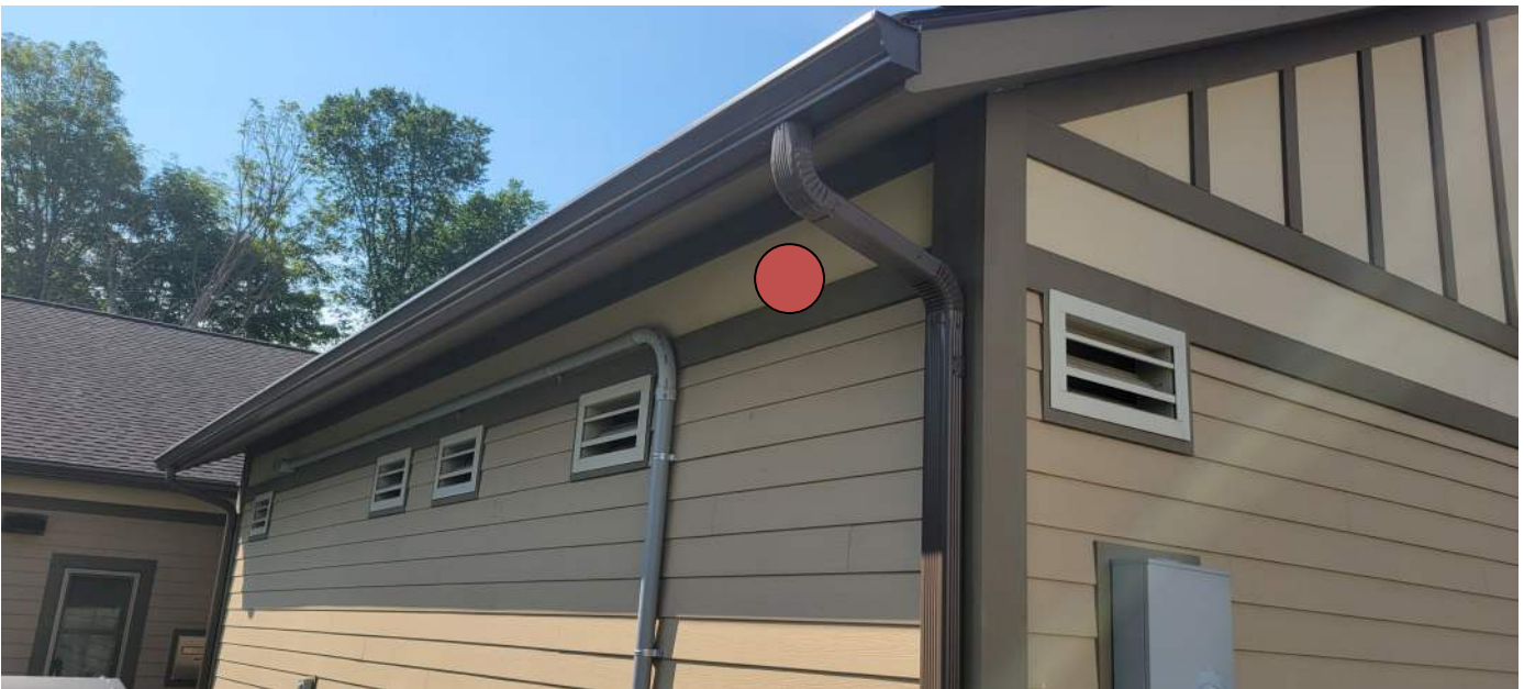
1 of 6 new camera locations Back of building near generator
