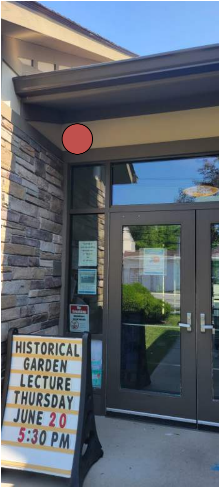
2 of 6 new camera locations Front of building, above main entrance
