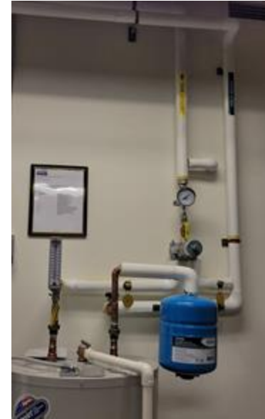
Well insulated pipes help to conserve energy
